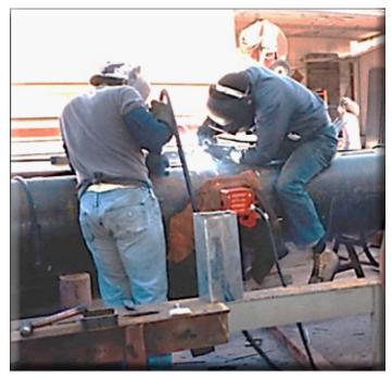
Expected weld distortion never occurred thanks to Meta-Lax weld conditioning. Navy inspectors were amazed at the quality and straightness.
