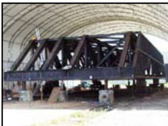
Bulkhead Dam Gate
